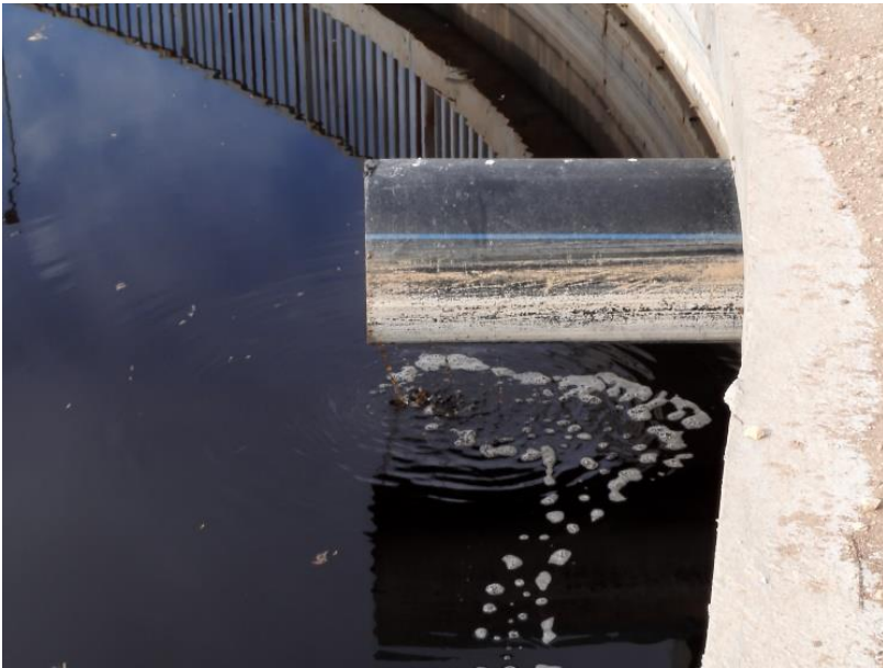
Figure 6. Leachate coming from the landfill cell drain
