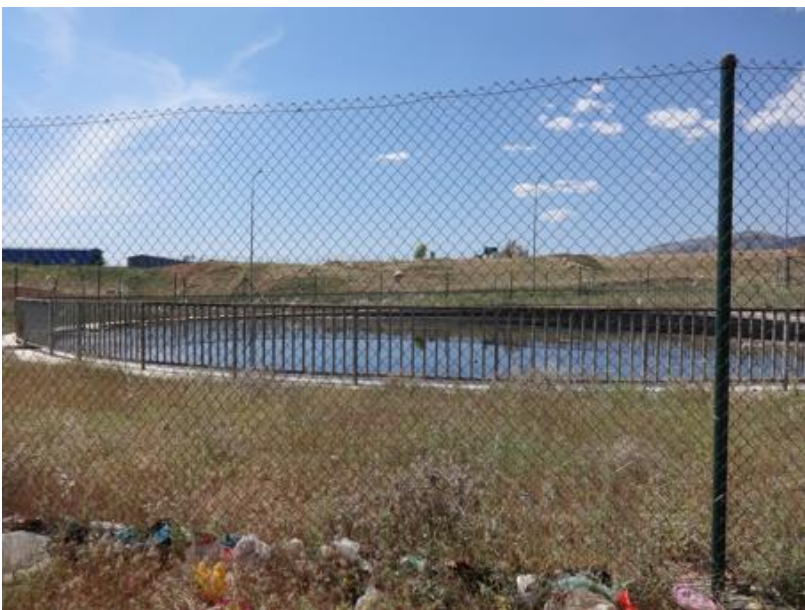
Figure 4: Leachate buffer tank
