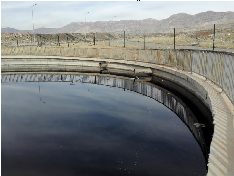
Figure 5. Existing leachate buffer tank (V=3,000m 3 )
